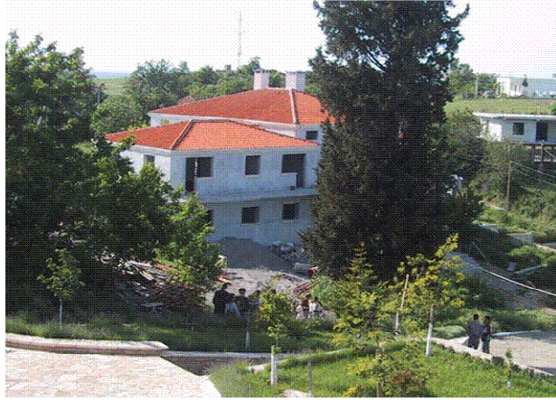
The new orphanage is almost complete.
